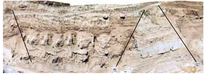
Figure 3. Local parallel faults influencing the block dimension in the Travertine Quarry
